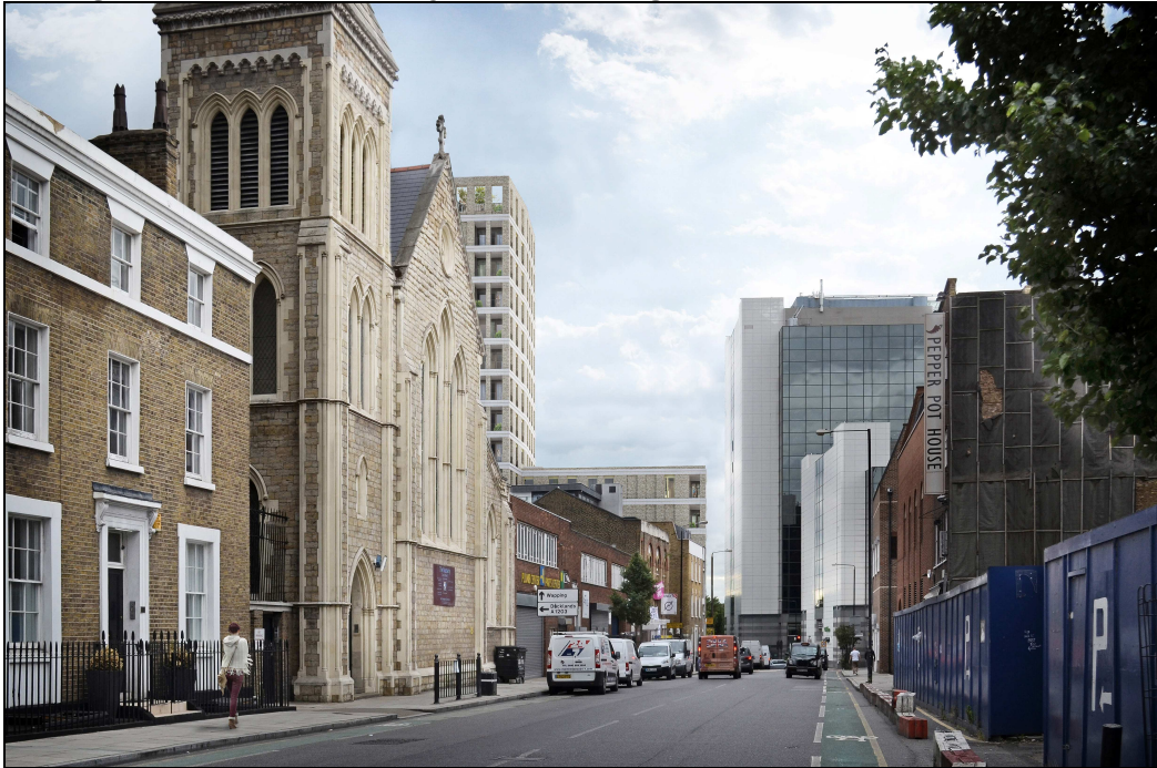
Figure 6: View south along Dock Street with the Grade II Listed Church in the Foreground and the Locally listed building at 15 Dock Street further down
